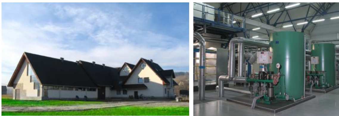
Figure 3.1 The peak load boiler house
