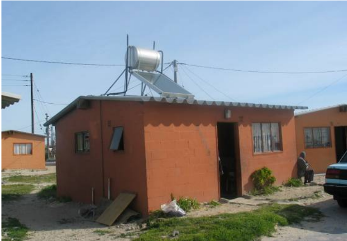
Figure 3.3 Social housing with subsidised solar water heater Source: City of Cape Town, 2007.
