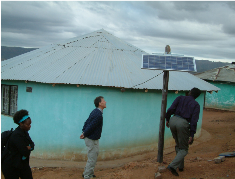
Figure 3.1 Solar home system mounted on a pole next to the house, as roof structures are often not suitable for supporting the system
