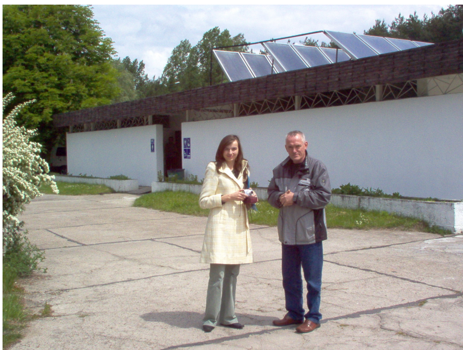
Figure 5.1 Solar installation at the camping site in Borki
