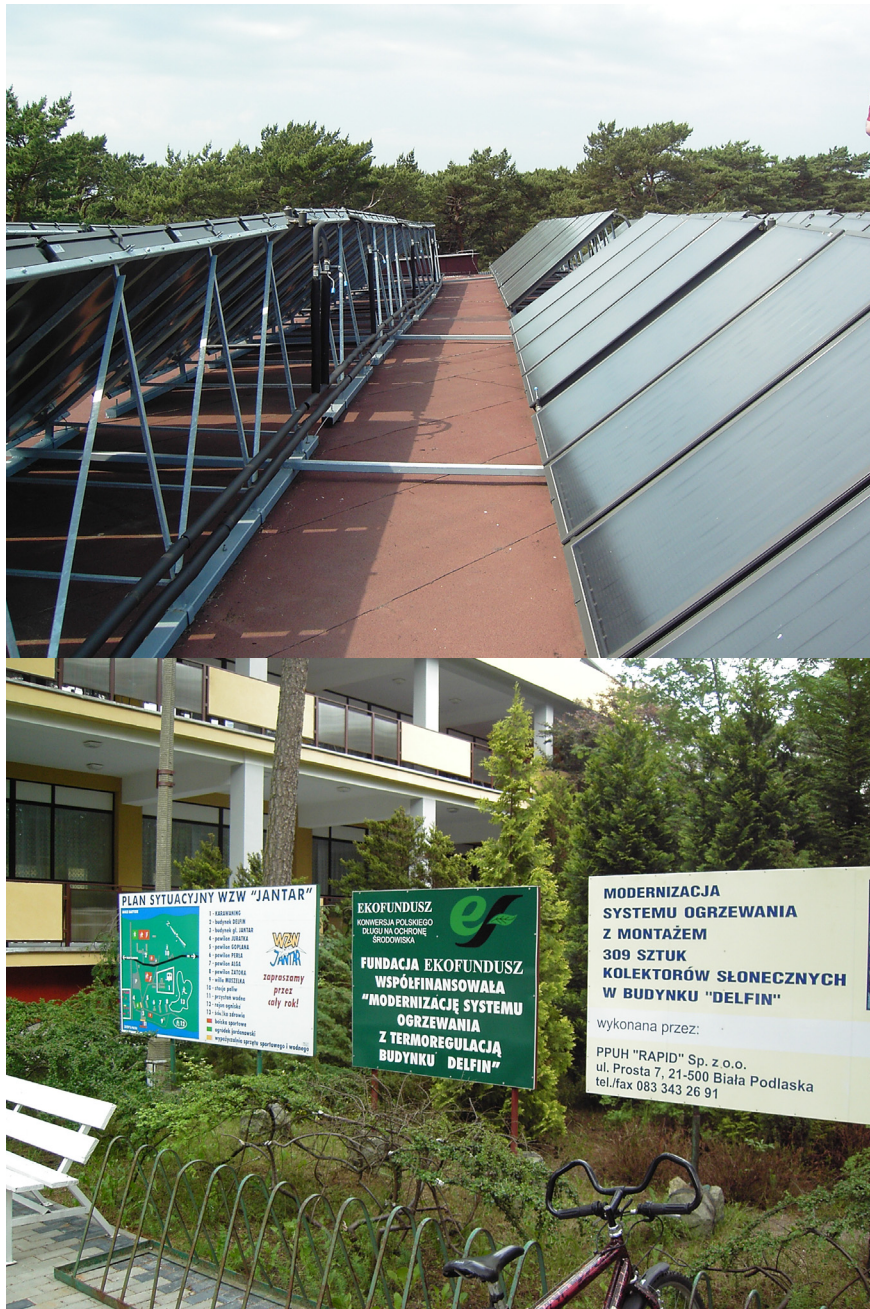
Figure 5.2 Solar installation at the holiday resort in Jurata
